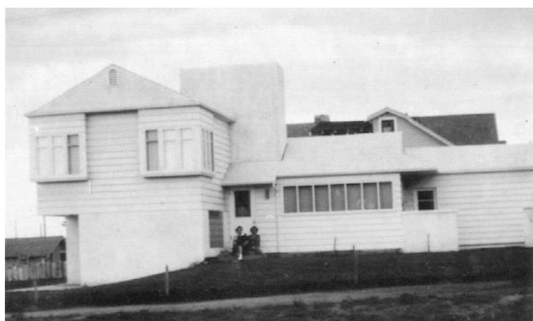
The Collier's $7500 House, shortly after its construction for the Brandley family.
