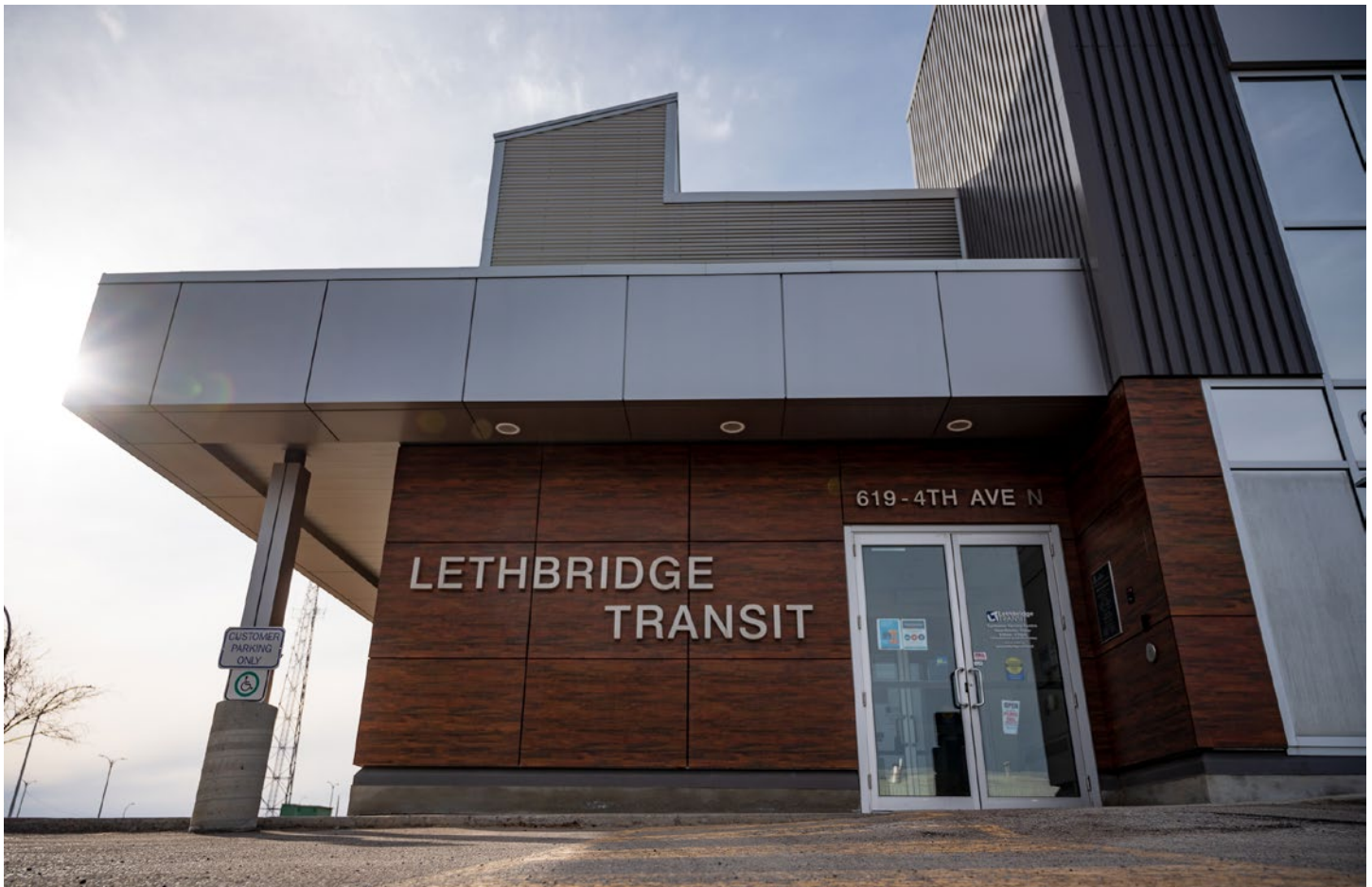
Lethbridge Transit Office Building
