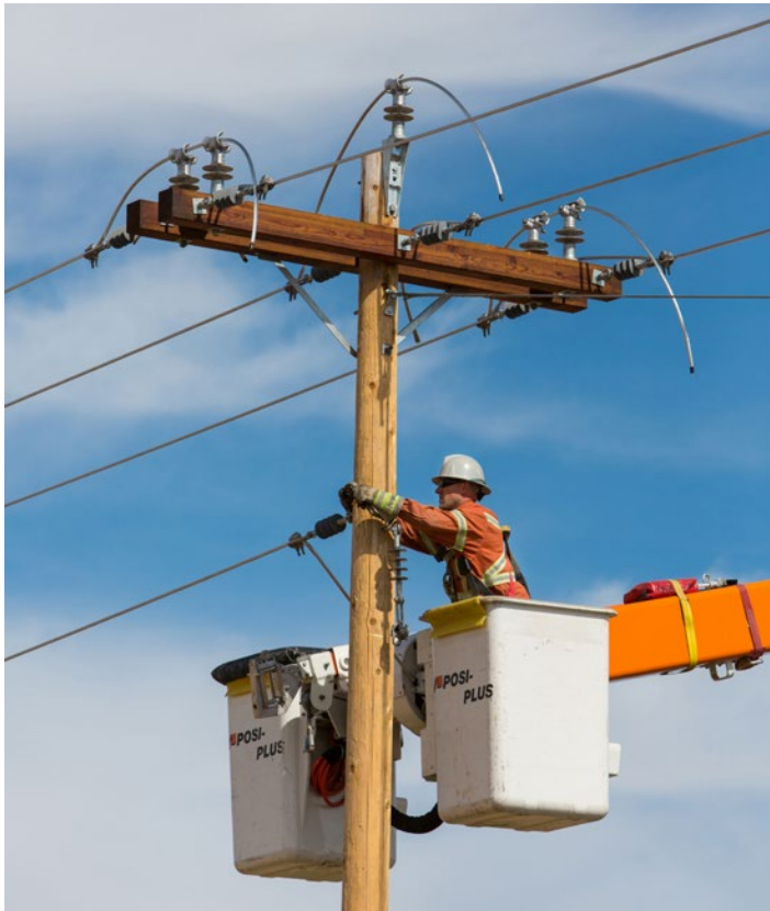
Lethbridge Electric Utility Worker
