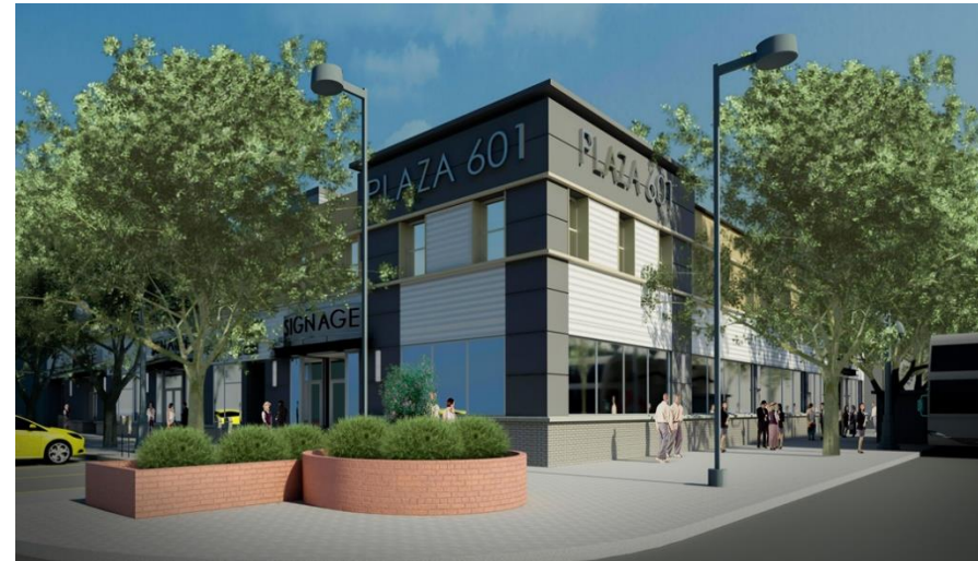
Suites at 601 Condo Project, Downtown Lethbridge
