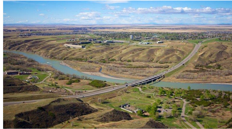
Main Crossing to Access West Lethbridge
