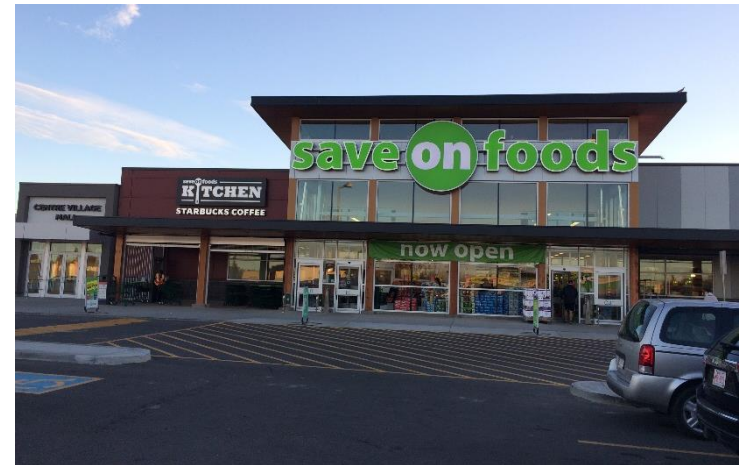
Centre Village Mall, north Lethbridge
