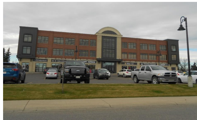
Southgate Station, south Lethbridge
