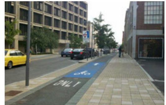
The cycle track remains level at driveway crossings, requiring turning vehicles to cross a steep apron to access parking.
