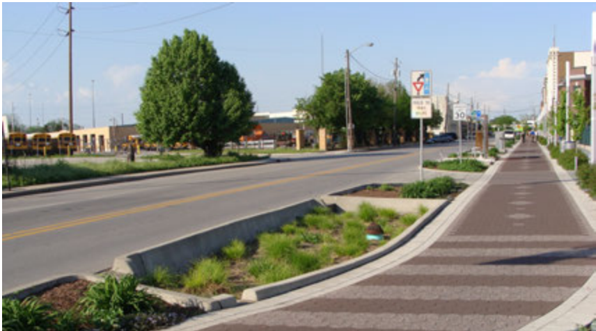
A protected bike lane provides separation from the adjacent roadway and includes treatments that increase cyclists visibility at conflict points.
