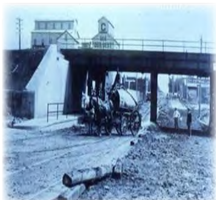
13 Street Underpass, built in 1915 to connect the north and south.
