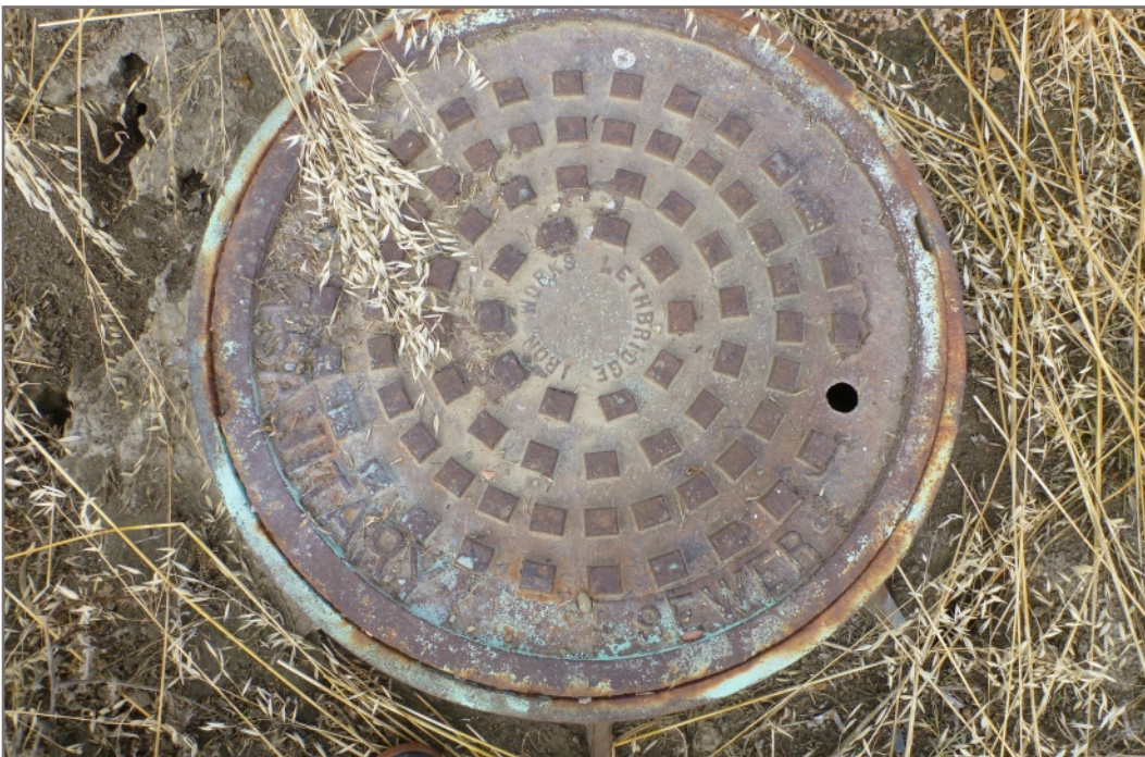
Photo 2: Sanitary Sewer 1 found within Suspected Wetland 1.
